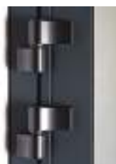
Paumelles et joint anti-pince doigts
